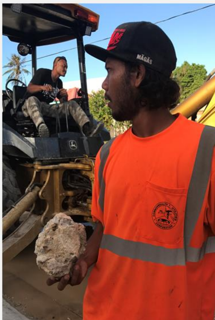
Backhoe operator Peter Attao removed dirt, including this rock, held by Water Operator Heirszan Martinez, to repair a break in a Garapan water line. Due to the vibrations of traffic, rocks can shift under the roads and sometimes move against water or sewer lines. Constant pressure from a rock eventually causes a water line to break. CUC inspects water and sewer line construction to ensure that the lines are surrounded by the proper materials to prevent future breaks in the water line.
