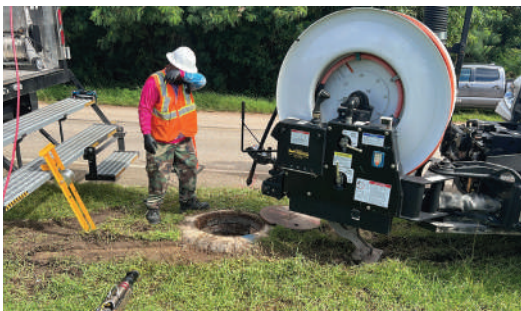
Wastewater Grout CCTV Inspection Truck
