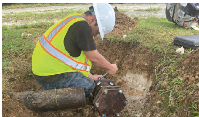
CUC Rota Water Operator Jesse Lizama works to cap an old 6-inch waterline pipe to help minimize water loss, strengthen system operations, and support reliable water service.
