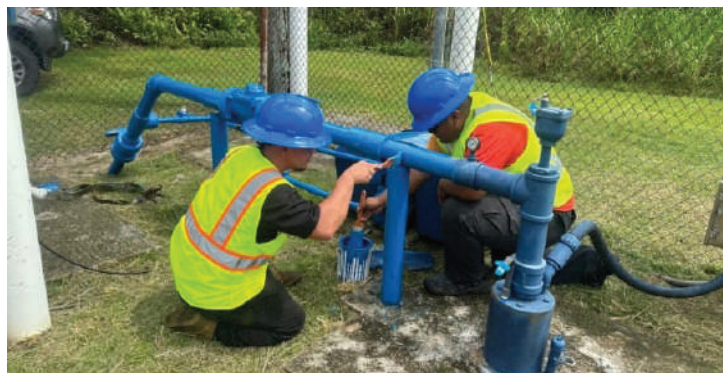
CUC Rota Water Operators Austin Lizama and Poly Jon Manglona perform routine maintenance by painting water wells to help preserve infrastructure and ensure reliable system operations.
