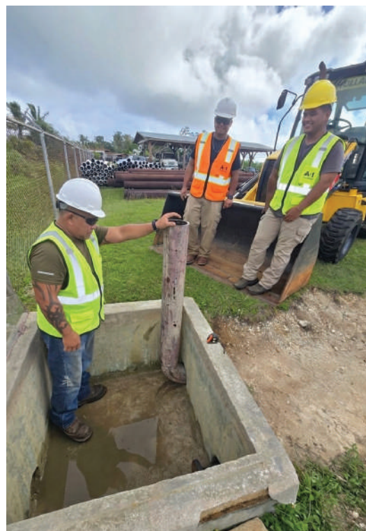
From left to right: Peter Taitano, Peter Mendiola, and Poly Jon Manglona, CUC Rota Water Operators, work on upgrading the overflow pipe at the 500K Ginalangan Water Reservoir as part of ongoing efforts to improve water system reliability and service for the Rota community.
