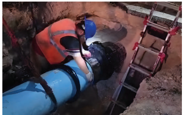
In February 2026, CUC Saipan Water Operators worked tirelessly around the clock to repair a mainline leak, dedicating a full day and continuing into the early morning hours to restore service. The repair was successfully completed at 3:30 a.m., reflecting the team's unwavering commitment to keeping water systems running for the community.
