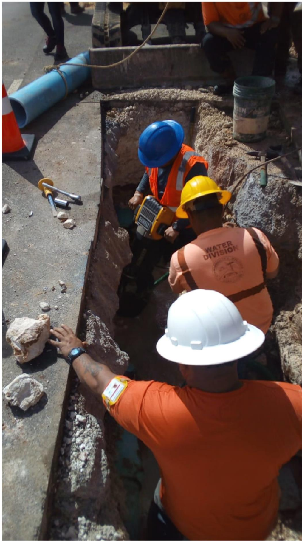
Peter Taitano, CUC Rota (bottom), Ralph Ascano, CUC Saipan (middle), and Mike Benavente, Guam Waterworks Authority (top) work together to remove rocks under an 8-inch waterline. CUC thanks the many operators from our neighbor islands of Rota and Guam who helped CUC Saipan and Tinian restore water services after Super Typhoon Yutu.
